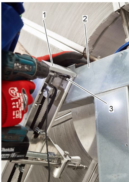
Fig. 31: Fasten the cleaning rail
