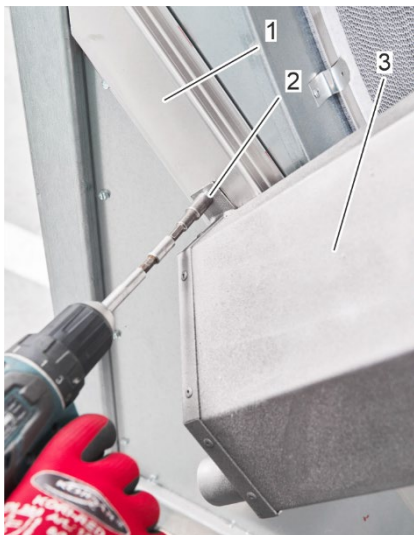
Fig. 53: Fasten the drip pan
