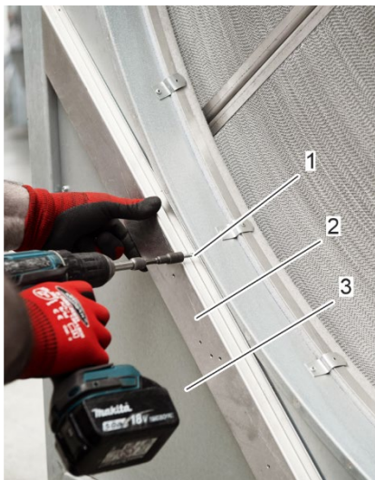
Fig. 23: Bolt crossbeam
