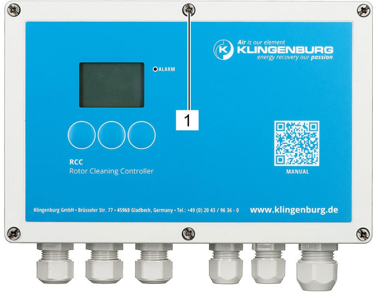
Fig. 82: Housing screws
