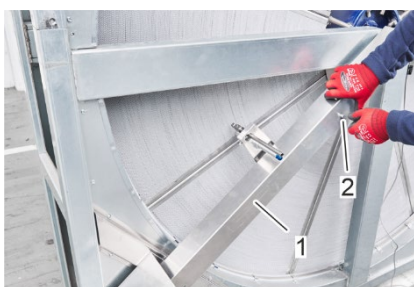
Fig. 56: Fasten the cleaning rail cover
